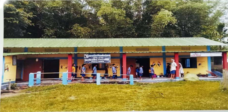
Name of Scheme:- Infrastructure Development work at Khamtighat Kasomari Hatigarh L.P. School Name of G.P.:- Jokai G.P, Under Barbaruah Dev. Block Estimated Amount:- 13,41,817/-
