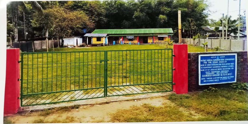
Name of Scheme:- Infrastructure Development work at Khamtighat Kasomari Hatigarh L.P. School Name of G.P.:- Jokai G.P, Under Barbaruah Dev. Block Estimated Amount:- 13,41,817/-
